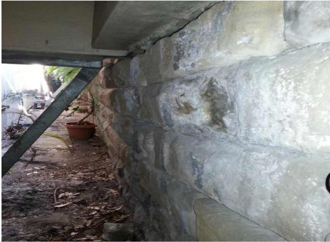
Photo 1 & 2 – Bulging and tilting sandstone block retaining wall. Steel brackets installed by Owners Corporation to support suspended access to building
