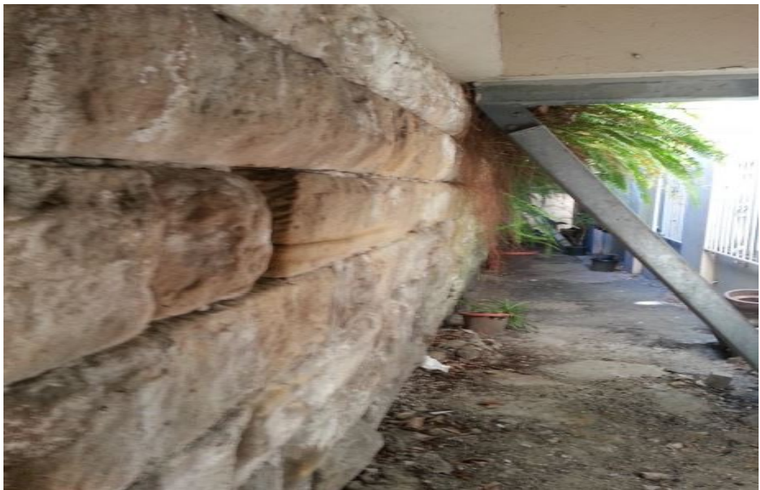
Photo 1 & 2 – Bulging and tilting sandstone block retaining wall. Steel brackets installed by Owners Corporation to support suspended access to building
